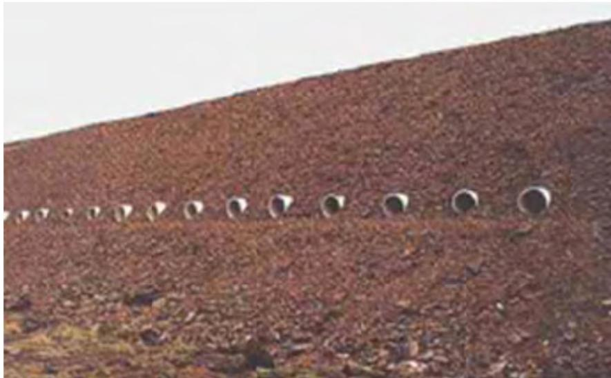
**Figure 3:** Ventilation Pipe Embankments
